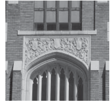
Detail of entryway, Old High School Building.
