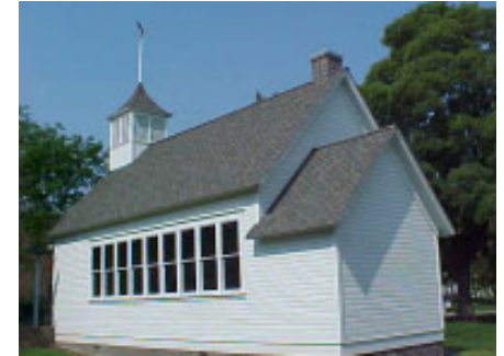
The Jore School at its new location on the EWU campus, 2002. Photo courtesy Cheney Planning Department.
