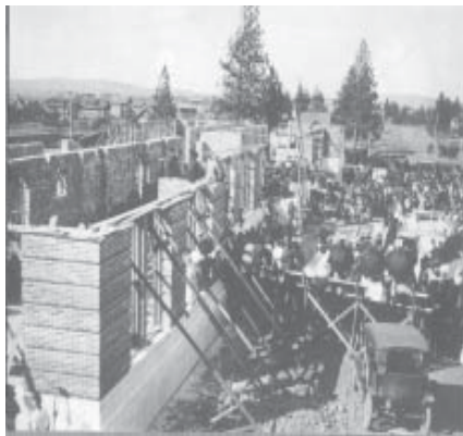
Senior Hall construction, 19__ (?). Photo courtesy Cheney Tilicum Museum.
