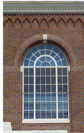
Window Detail, Hargreaves Hall. Photo courtesy Cheney Planning Department.
