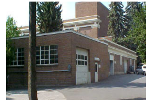
Plant Utilities Building. Photo courtesy Cheney Planning Department.
