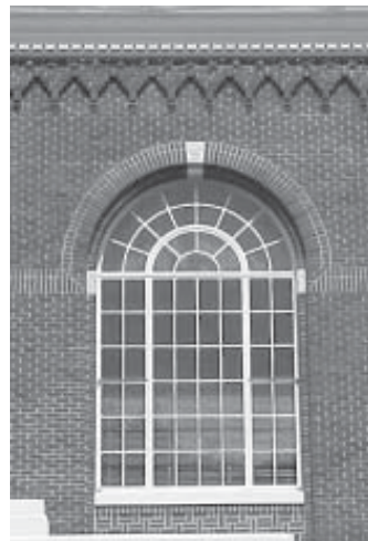
Window Detail, Hargreaves Hall. Photo courtesy Cheney Planning Department.
