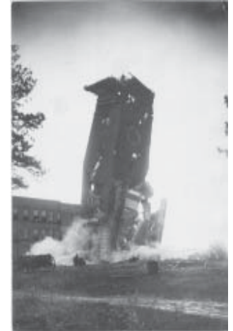
Destruction of the old Normal School tower following the fire of 1912. Photo courtesy Cheney Historical Museum.
