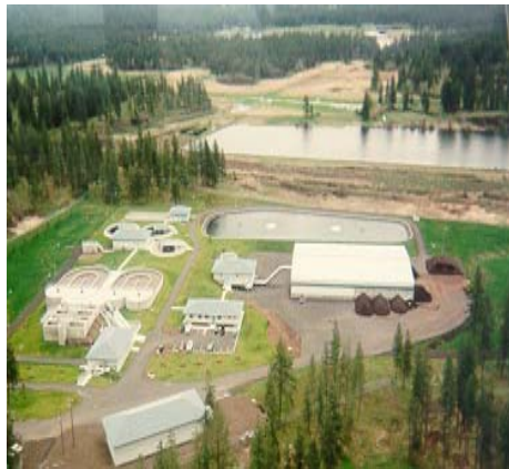
Aerial View of the City of Cheney Wastewater Treatment and Reclamation Plant
