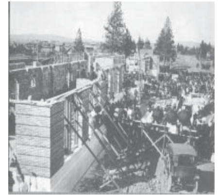
Senior Hall construction, 1918. Photo courtesy Cheney Historical Museum.
